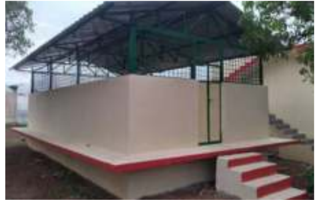
Fig. 126. Spices storage Structure, UHS, Bagalkot
