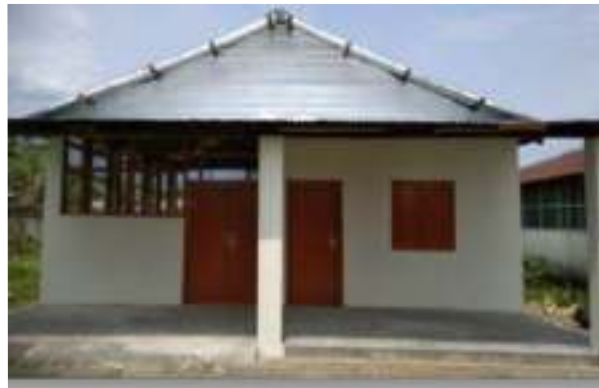
Fig. 127. Turmeric Storage structure at CAU, Pasighat
