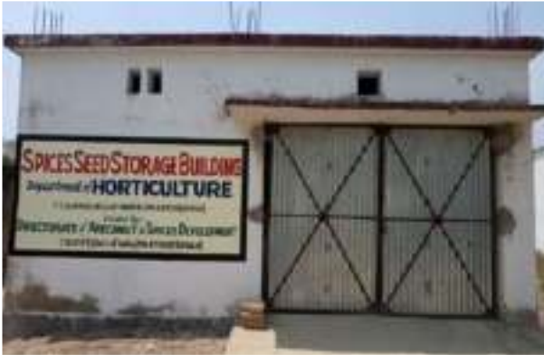
Fig. 125. Storage structure for Turmeric at Rajendra Agri University, Bihar
