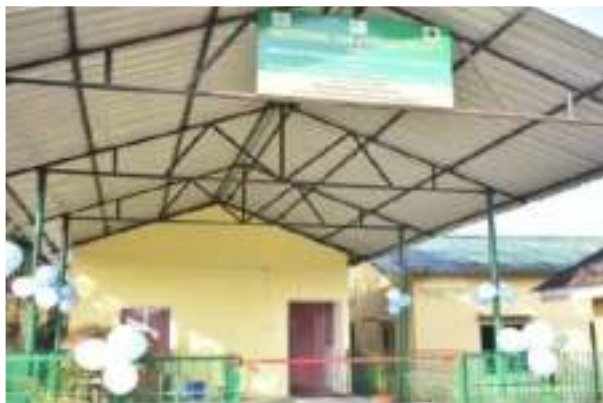
Fig. 124. Turmeric storage structure established at AU, Assam
